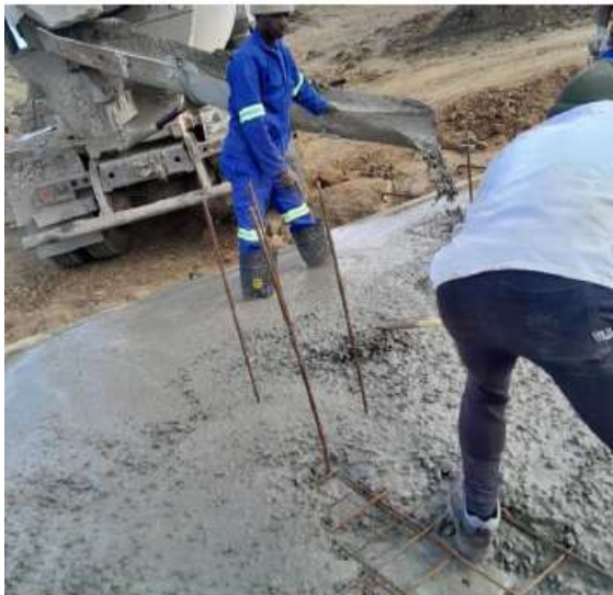
Pouring of concrete for causeway
