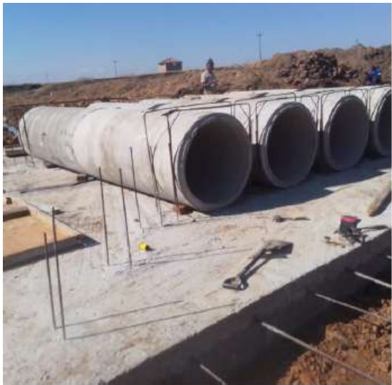
Preparation for a top slab- causeway
